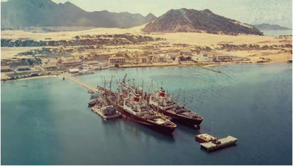
When the 35th Engineer Group arrived at Cam Ranh Bay, the only deep-draft pier was the one built by RMK in 1964.
